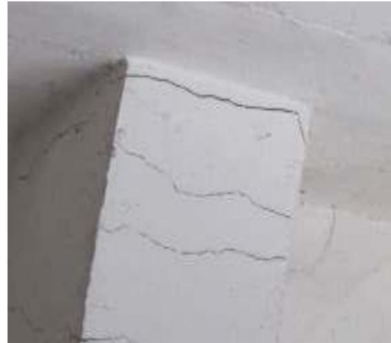
3) 柱构件纵向裂缝
